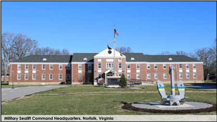
Military Sealift Command Headquarters, Norfolk, Virginia
